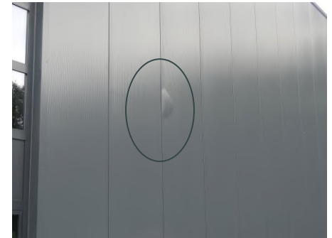
Blistering of lightweight sandwich panels
